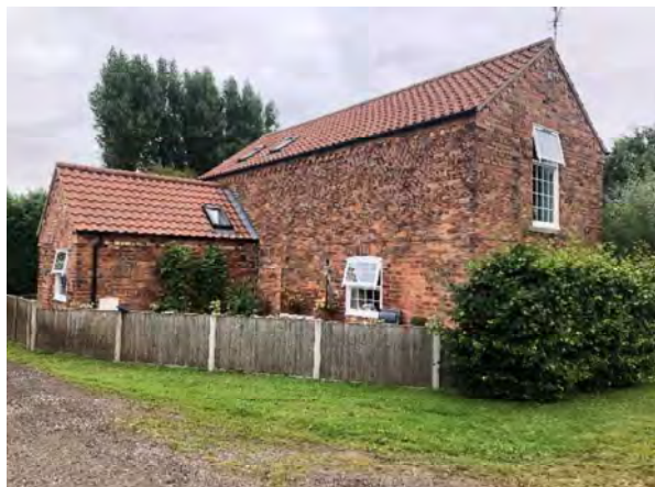
Image .06 – View from within the site looking East.
